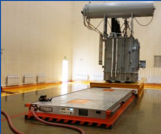
Mega Voltage Transformer Transport
